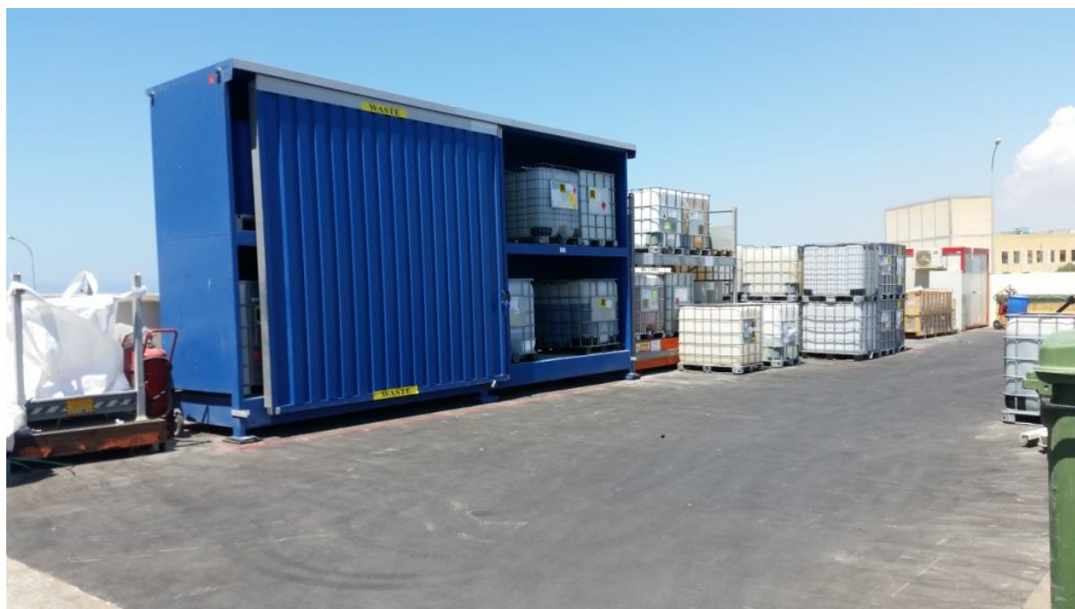
Figure 4.1: New temporary waste storage area showing main containment system
